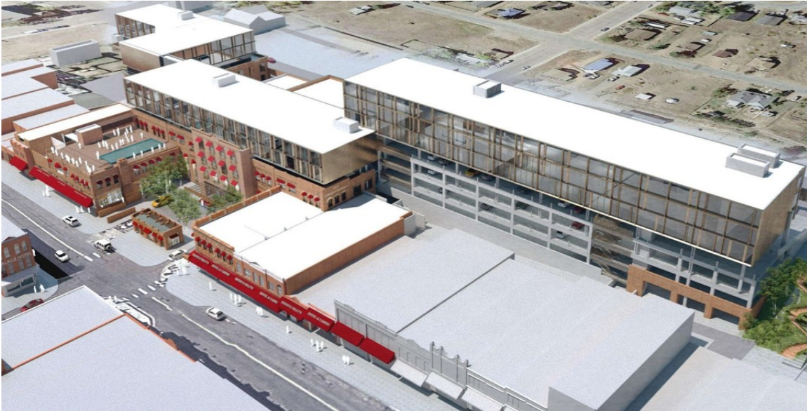
Construction continues at Chamonix Casino Hotel, a new luxury gaming destination anticipated to open in mid-2023 in Cripple Creek, Colorado.
